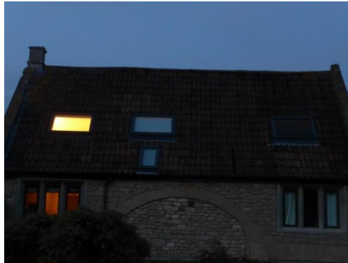
Left to right : (1) no blind; (2) internal venetian blind; (3) internal and external blind
